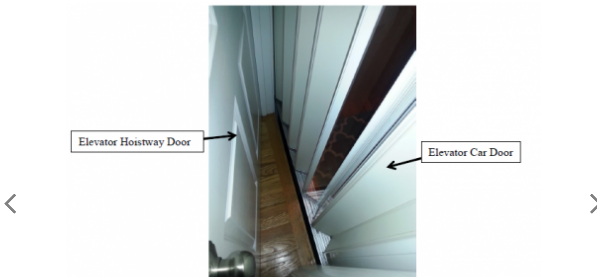
Figure 1. Typical Residential Elevator with Swinging Hoistway Door and Accordion Car Door
