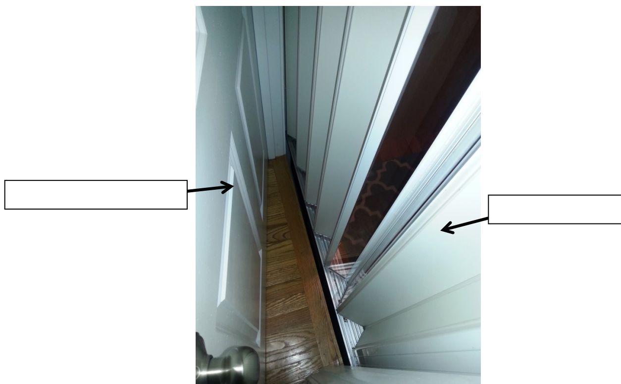
Figure 2. Typical Residential Elevator with Swinging Hoistway Door and Accordion Car Door
