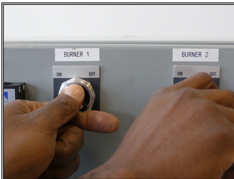
Figure 3. Step 9 Turn burner switches to "ON" position.
