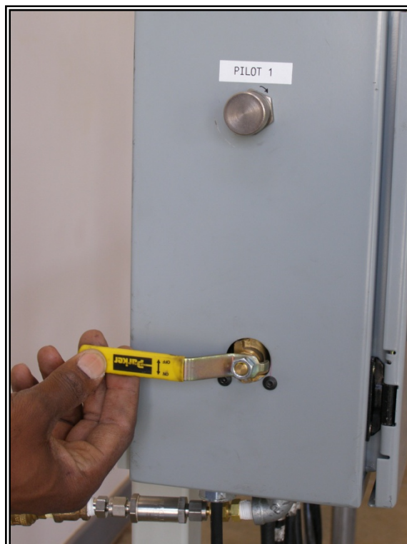
Figure 2. Step 6 Open the ball valves for both burner pilots.
