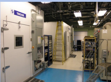
Combustion Products Test Lab
