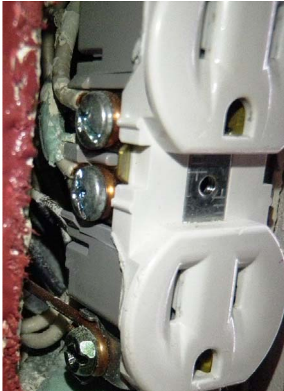
Figure A4. Receptacle wired via WBS terminals.
