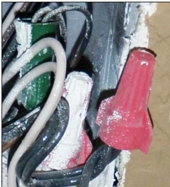
Figure A5. Twist-on splicing connectors.
