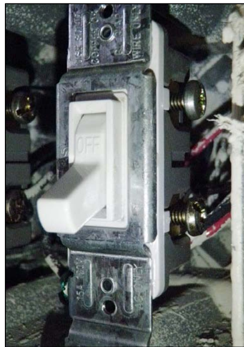
Figure A6. Back-wired switch.
