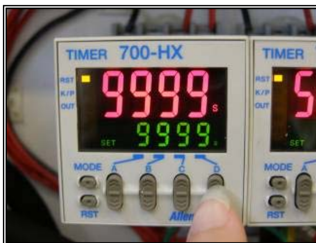
Figure 46. Step 5 Timer set to maximum time
