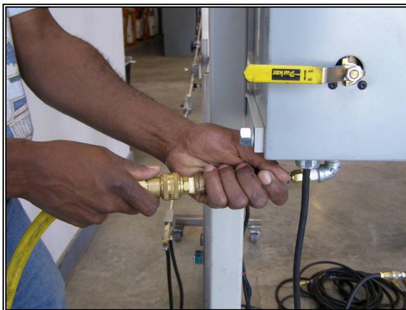
Figure 9. Step 2 Connect propane supply.
