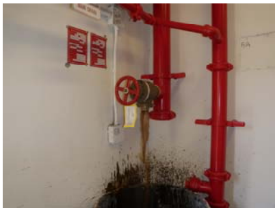
Figure 3 – System Drain
