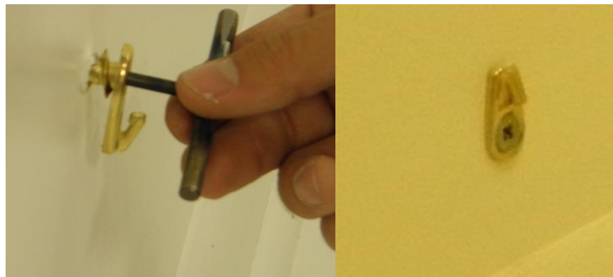
Figure 3. The drywall anchors were used to fix upside-down metal hooks to the wall.
