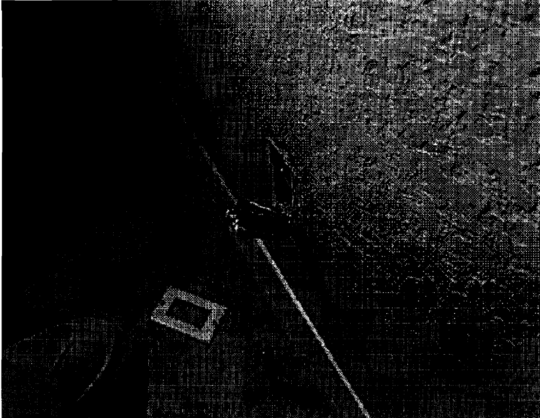
PHOTO 4 – View of an outlet in the bedroom where the ground wire turned black
