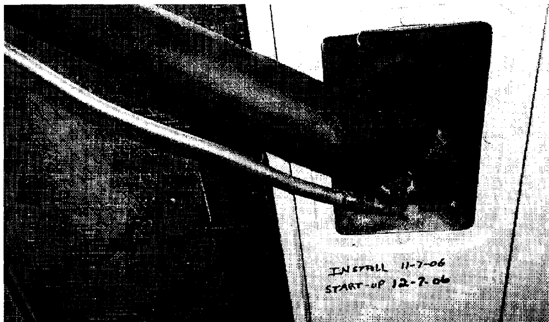
Exhibit 20 - Photo of blackened copper pipe outside of second floor air handler.
