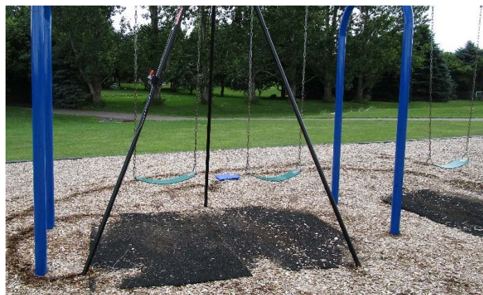
Figure 3. Rubber mats installed under the swing exit use zone region
