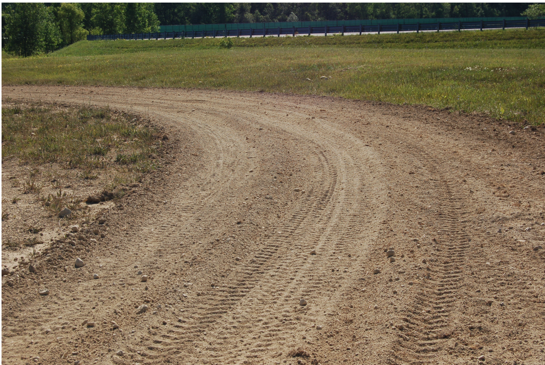
Figure 2: Prepared Dirt Surface after Several Tests were Completed
