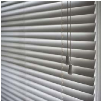
Figure 11 Horizontal Blind with Accessible Operating Cord
