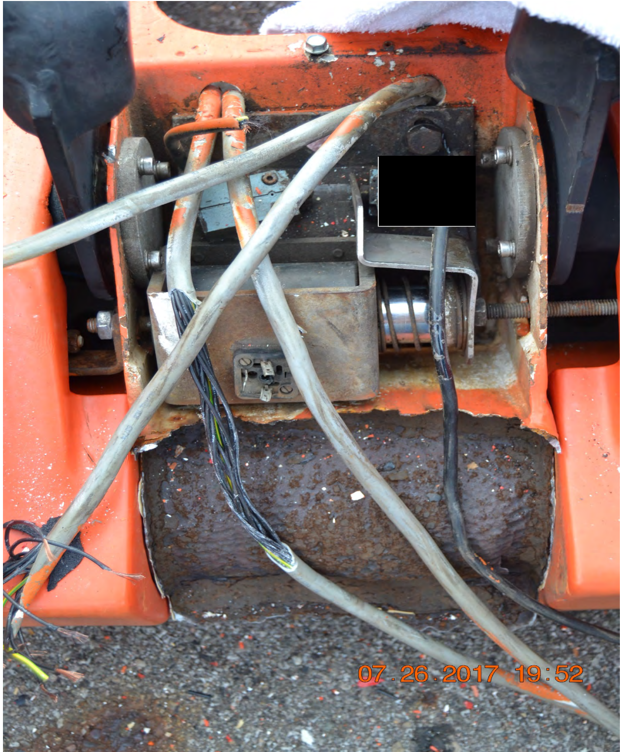
Photo #14 – Additional close up picture of the incident ride. Photo identifies the inside of the arm on the gondola that separated from the ride. Photograph taken by the [REDACTED] State Highway Patrol on July 26, 2017 after the incident.
