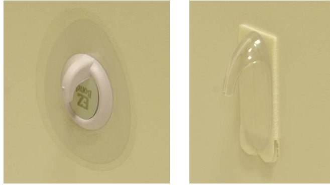
Figure 10. The plastic hooks are shown adhered to the drywall.
