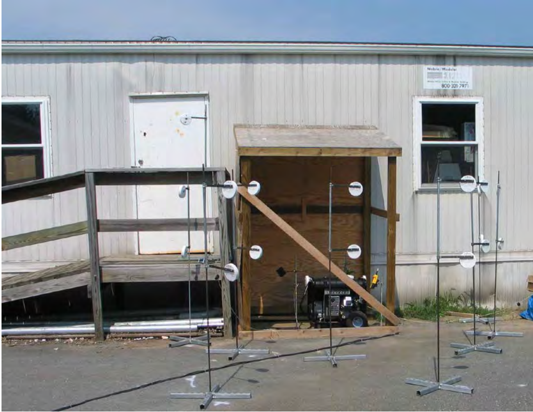
Figure A2: Two-Sided Roofed Area Adjacent to the TMS Building
